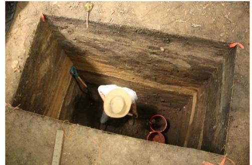
**What is wrong with this excavation?** It is not a staged photograph but a publicity shot of a real dig, used in a press article. For reference the hole measures 2m x 1m and was dug to a depth of 3m! It was not in the UK.
